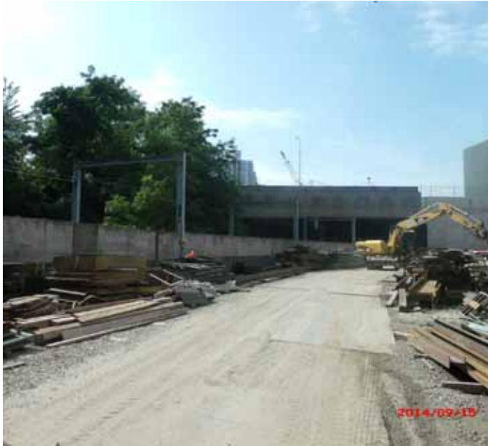
1 View looking south within Amtrak R.O.W.
