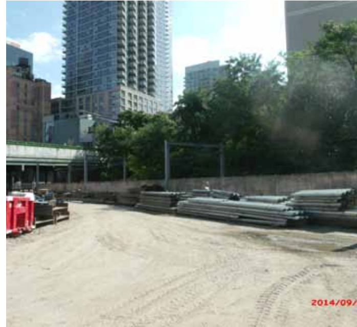
2 View looking northeast within Amtrak R.O.W.
